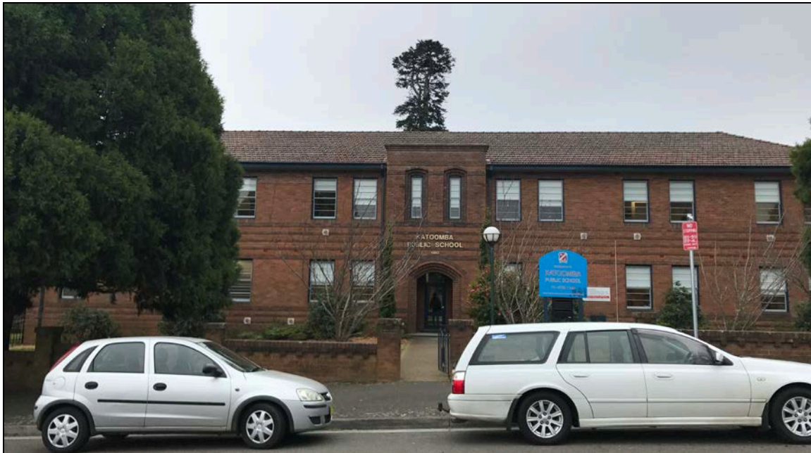
Figure 5: View of Katoomba Public School looking north from Merriwa Street
