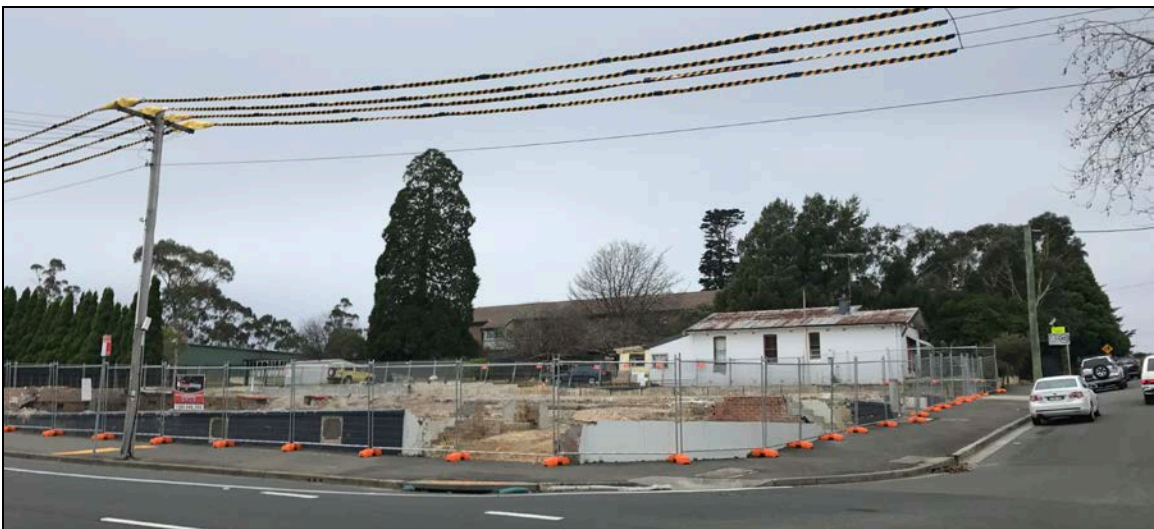
Figure 4: View of the site, with the remnants of the former RSL building in the foreground, looking north east from Lurline Street
