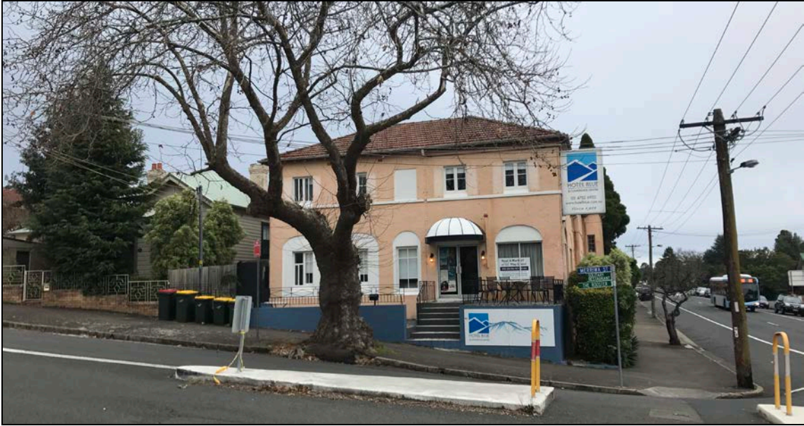
Figure 7: View of hotel to the south of the site, looking south east from Merriwa Street
